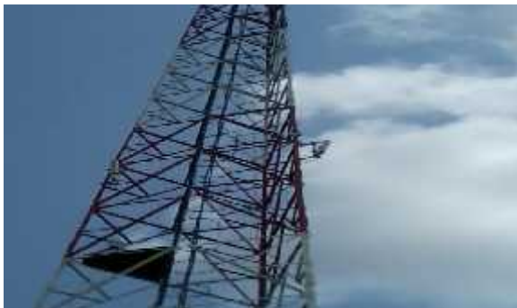
Figure7b: Antenna mast with Tranzeo and Wavion Radios
