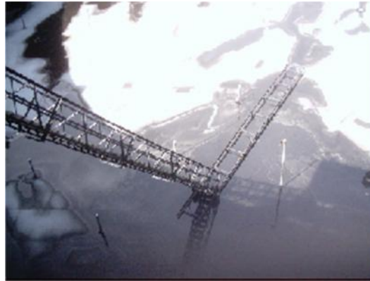
Figure 2: FRT Roof Access Ladder
