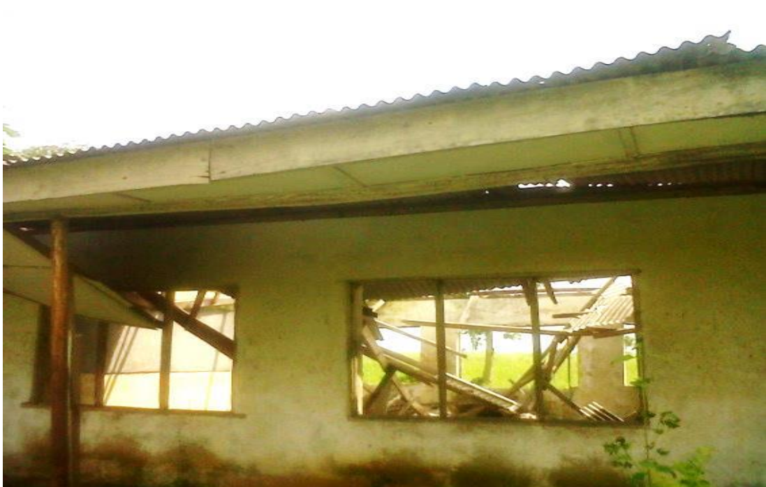
Plate 5.4: Deteriorated ROOFCO
