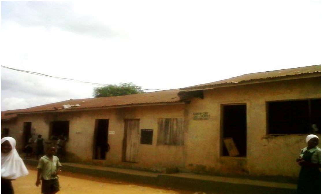
Plate 5.5: Rusted Roofing Sheets in ROOFCO
