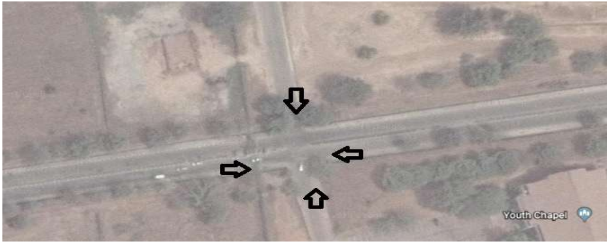
Figure 2: A Cross Intersection at the Entrance of Covenant University, Nigeria
