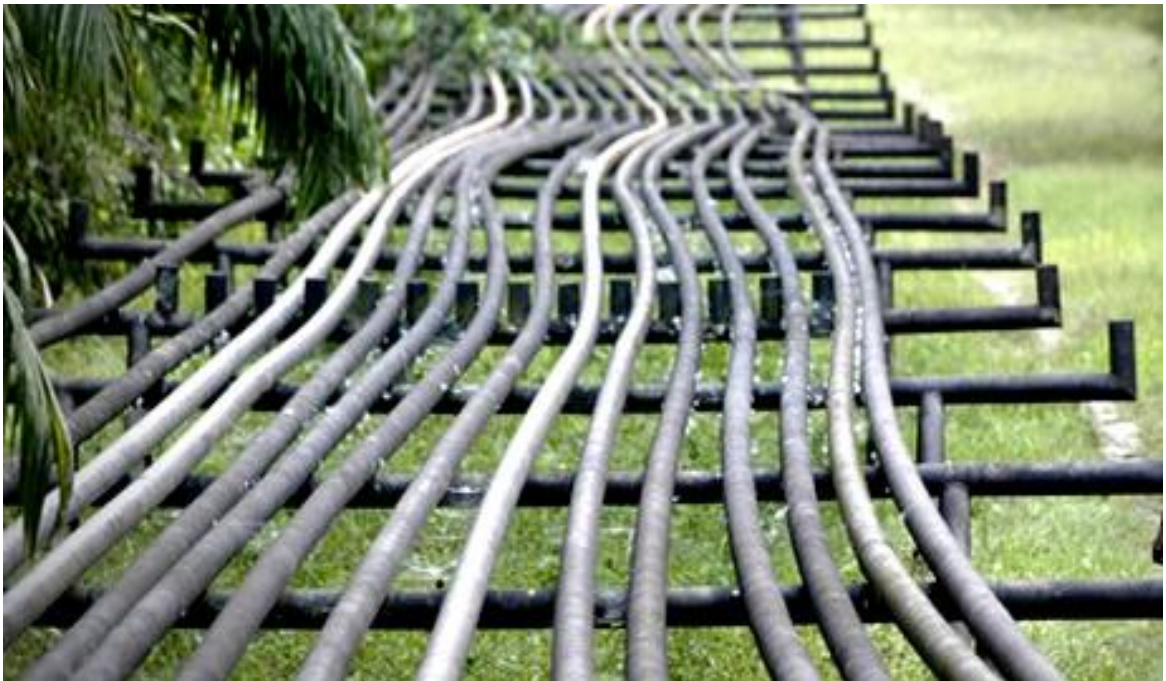
Fig. 4.5 A Maze of Oil Pipelines in Bayelsa State Source: Field Survey (2011)
