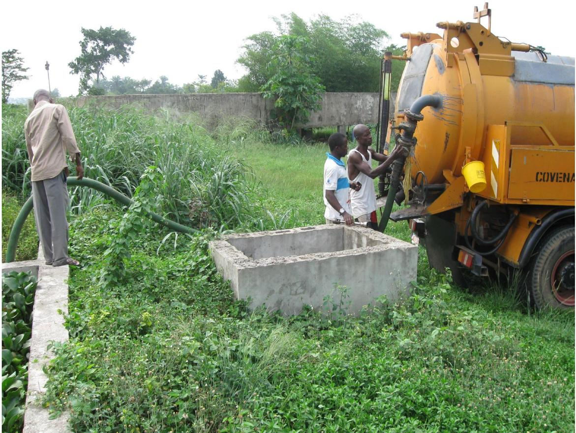
Plate 3.1 Shows tanker dislodging wastewater into the treatment chamber
