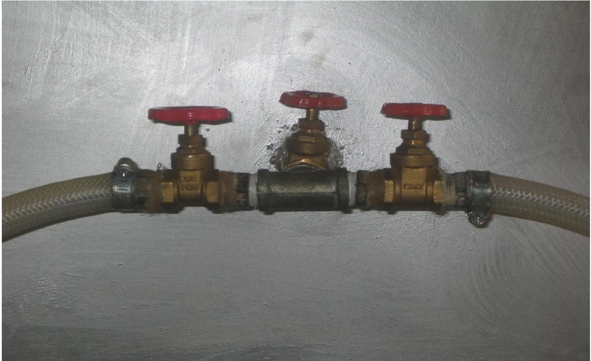
**Plate 3.15** Control valves screwed to position for wastewater flow
