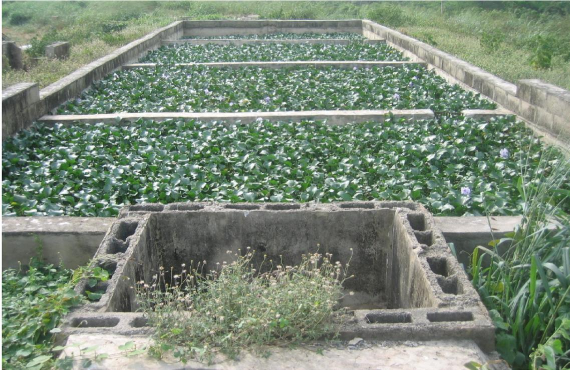
Plate 3.2 The water hyacinth reed beds showing baffle arrangement at opposing edges.
