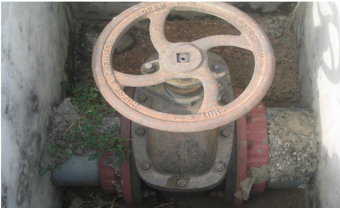
Plate 3.3 The inlet compartment showing gate valve
