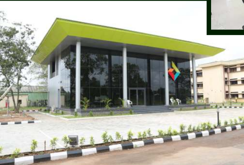
Frontal left side view of the Diamond Bank Building
