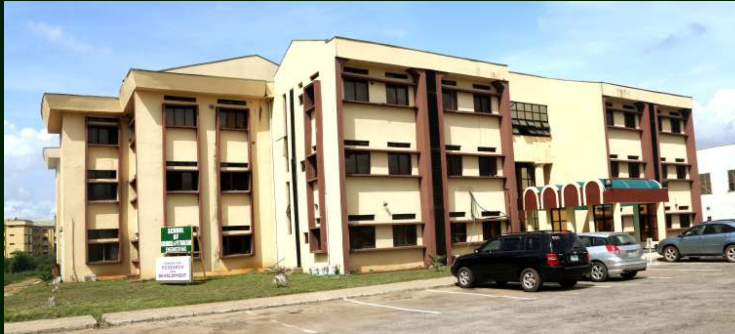
Front view of the Petroleum Engineering Building
