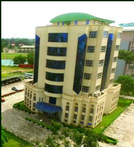
High elevation view of Senate Building
