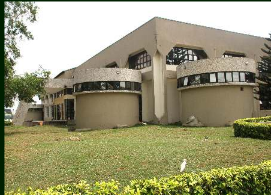
A side view of the Cafeteria 2 Building
