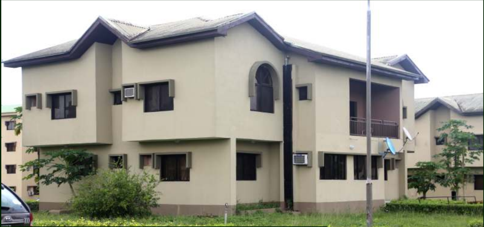
A duplex building in the Professors' Village
