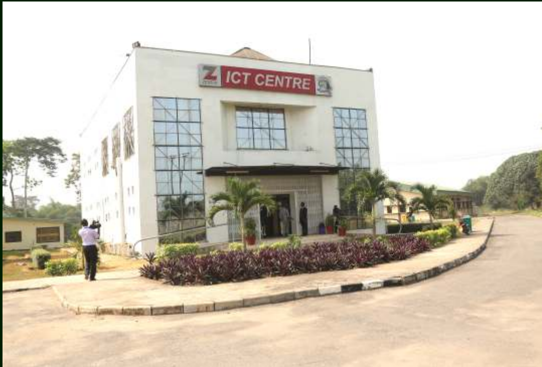
Front view of the ICT Centre donated by Zenith Bank
