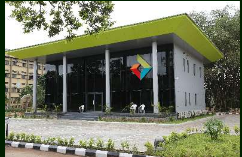
Frontal right side view of the Diamond Bank Building
