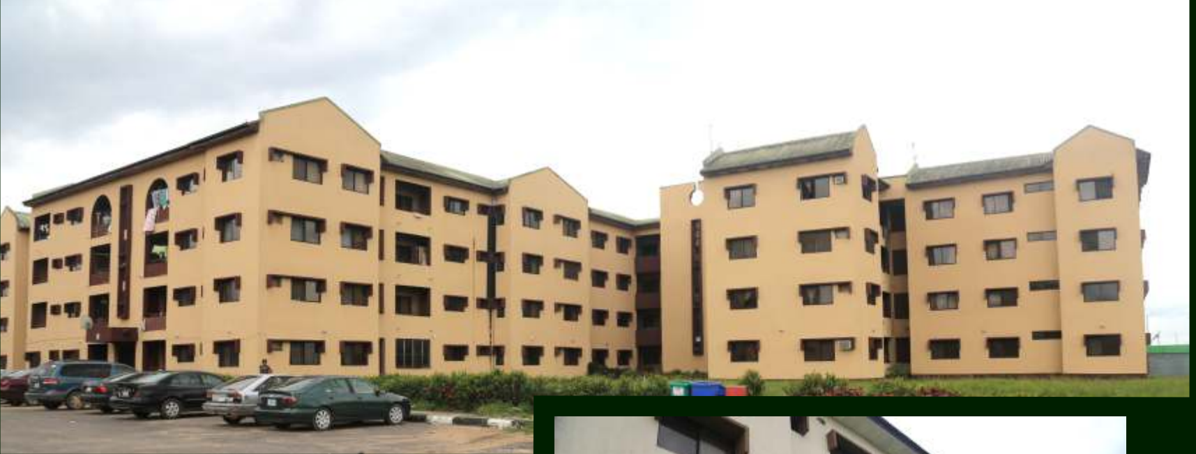
Long view of Old PG Quarters
