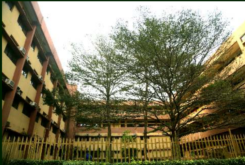
Side views of CLDS/CBSS Building showing trees
