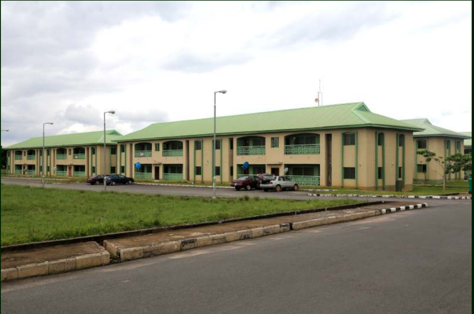
New rows of 2-Bedroom flats at the Covenant University New Estate
