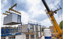
Fig 1: Installation of Modular Housing Source: Lawrence (2017).
