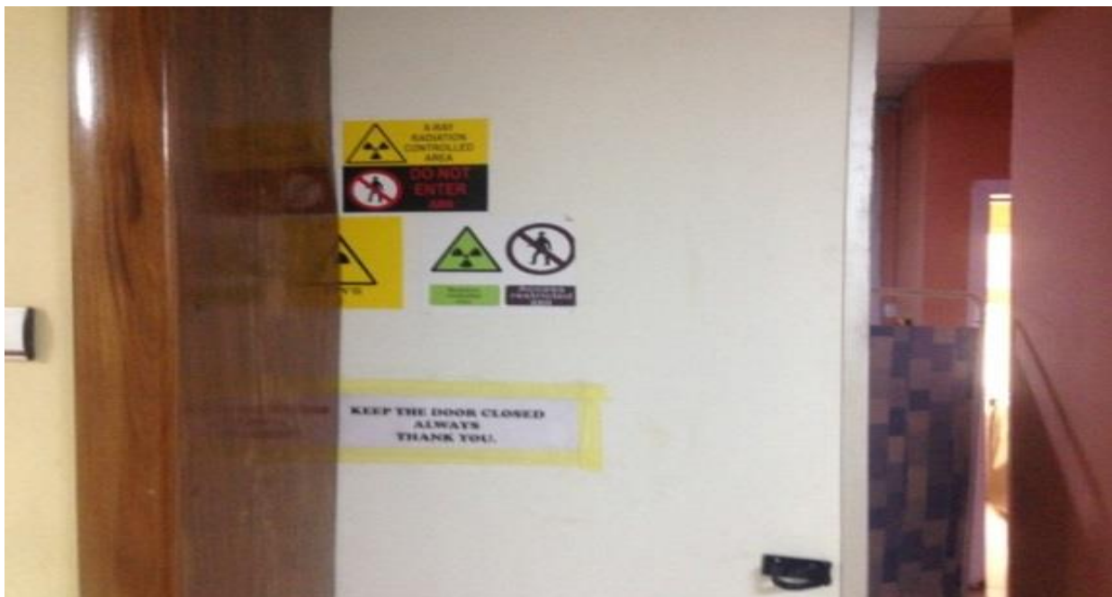
Plate 11: Lead door leading to the x-ray room with danger signs on the surface of the door.
