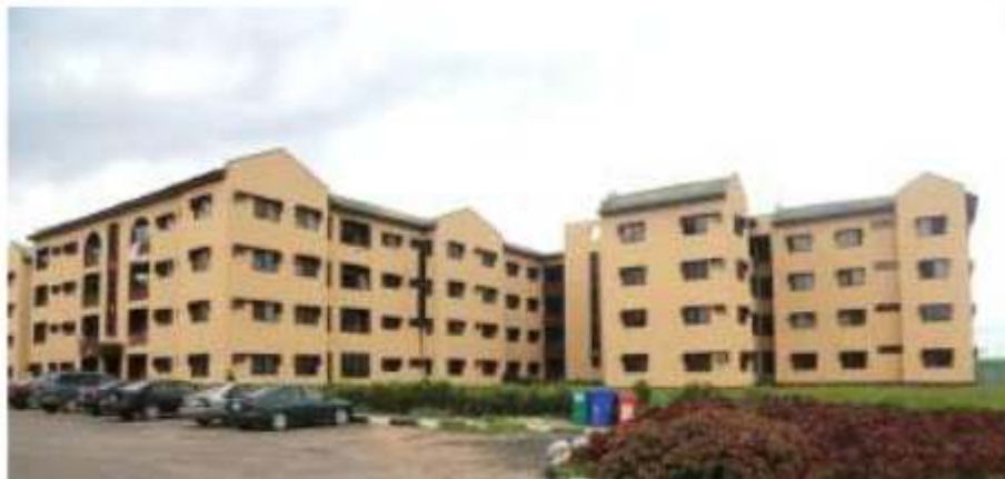
Staff Residential Complex
