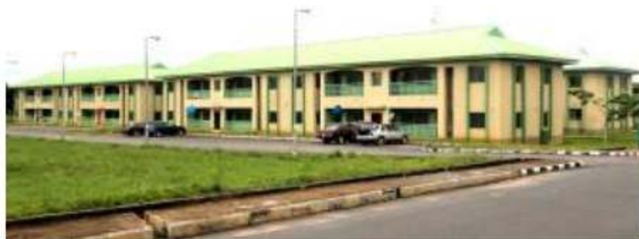
New Estate Staff Quarters
