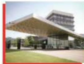
THE ESTATE GATE HOUSE
