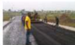
Resurfacing And Asphaltting Of Professors Village, Covenant University, Ota.
