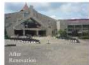
After Renovation Faith Tabernacle, Ota.
