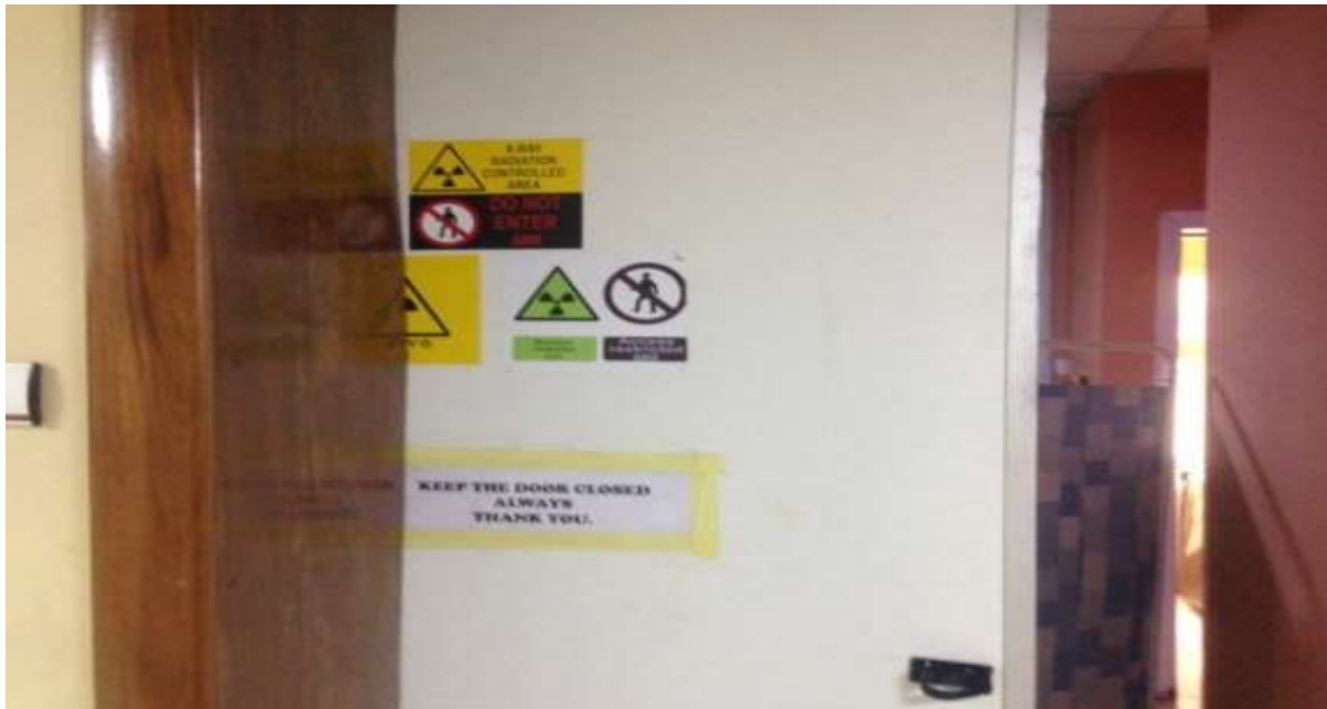
Plate 8: Lead door leading to the x-ray room with danger signs on the surface of the door.
