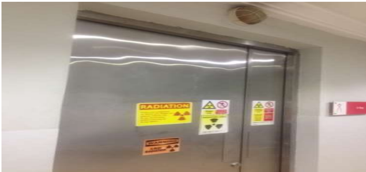
Plate 2: View of warning light above the door with danger signs on the surface of the door.
