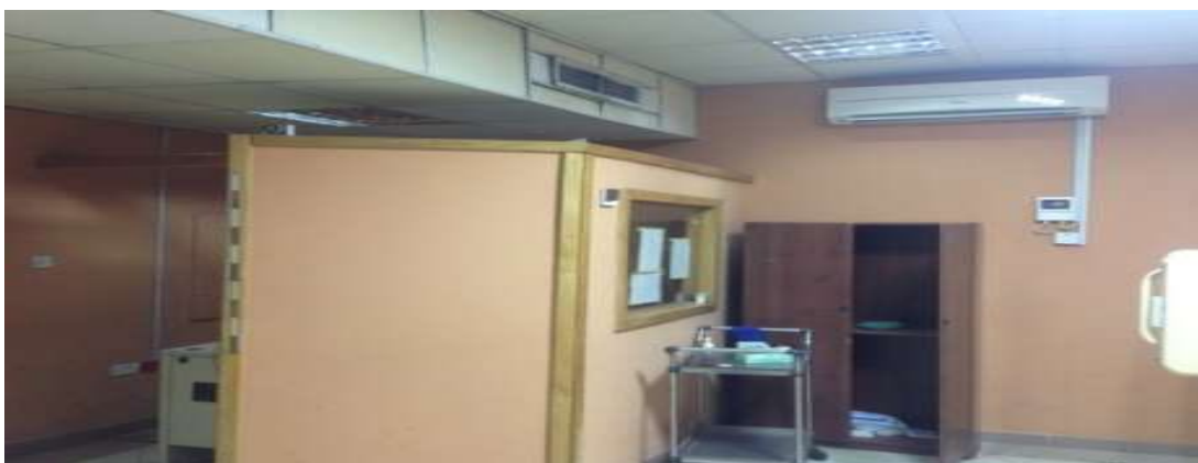
Plate 3: View of the protective cubicle in the x-ray room.
