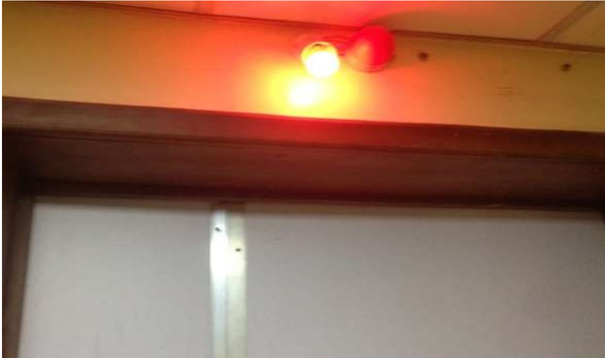
Plate 9: View showing danger signs on the entrance door leading into the radiology room.
