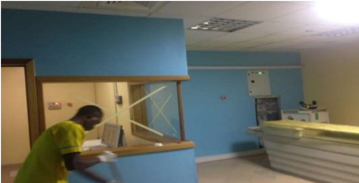
Plate 5: The operator control room with lead glass in the 16 slice CT room.
