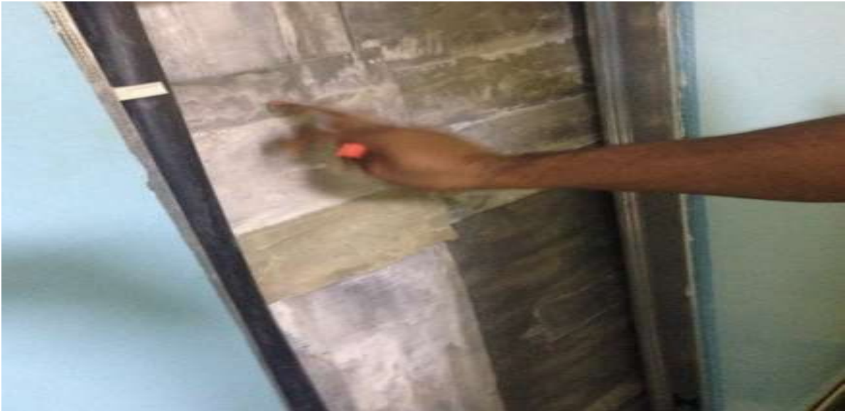
Plate 6: View of an uncovered lead lining in the 16-slice computed tomography room.
