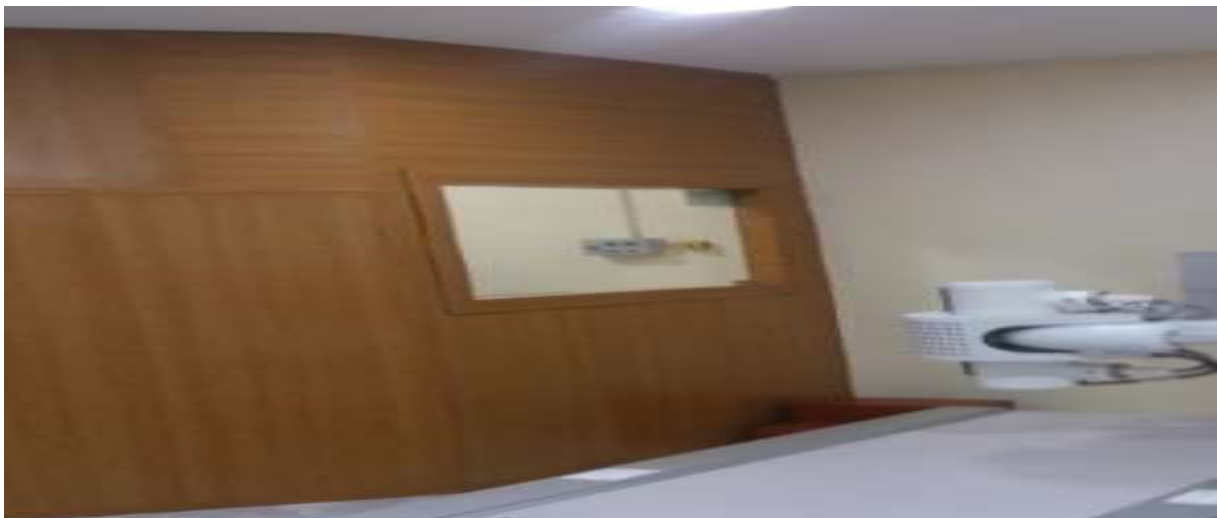
Plate 11: View of the protective cubicle in the x-ray room. Source: Author's field Study (2019)
