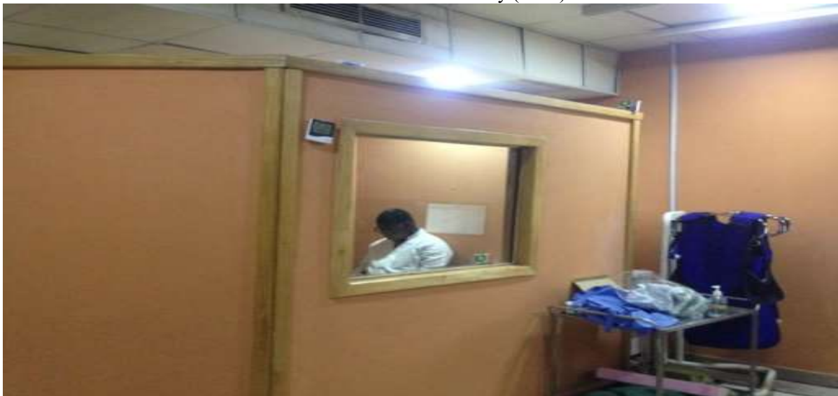
Plate 4: View of the protective cubicle in the fluoroscopy room.
