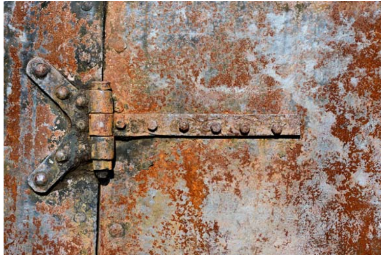
Figure 1: Corrosion of industrial infrastructure
