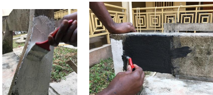
Figure 5. Physical tests on the two brand of paint products
