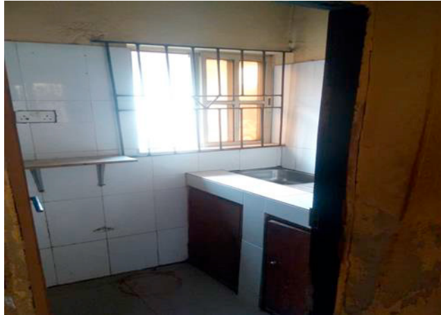
Fig. 1. Residential building in Ota
