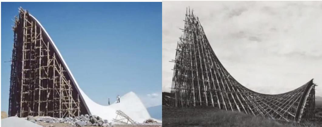
Plate 3. 13: Hyperbolic paraboloid thin-shell structure can be casted on straight surfaces
