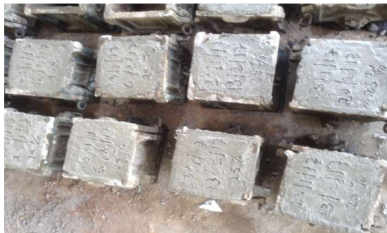
Figure 1. Moulding batch of WMD Concrete
