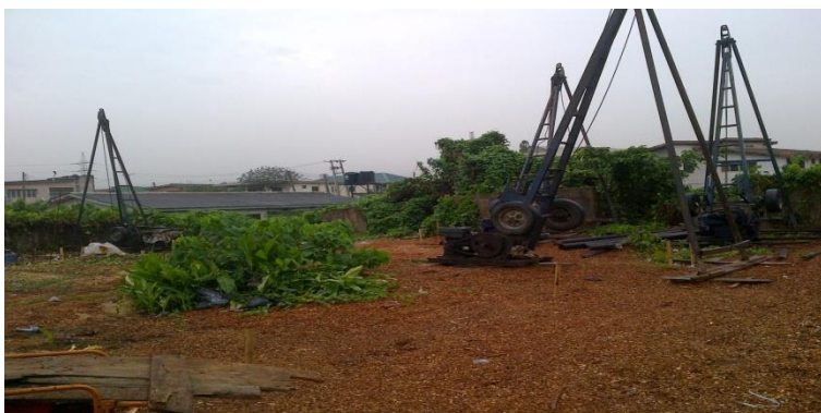
Figure 3: Pile driving machines in place
