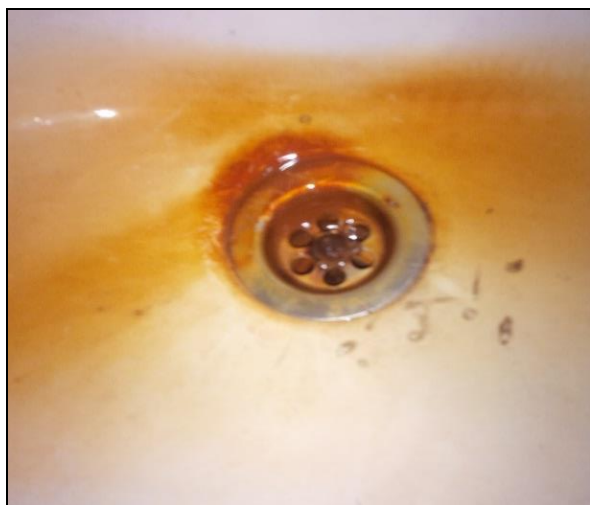
Fig. 1: Iron stained wash hand basin in a covenant university residence
