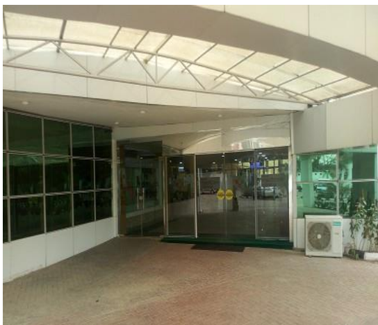
Plate 15: Main Entrance Porch View
