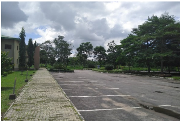
Figure 11. Side view of the Building with Adequate Vehicular Manoeuvring
