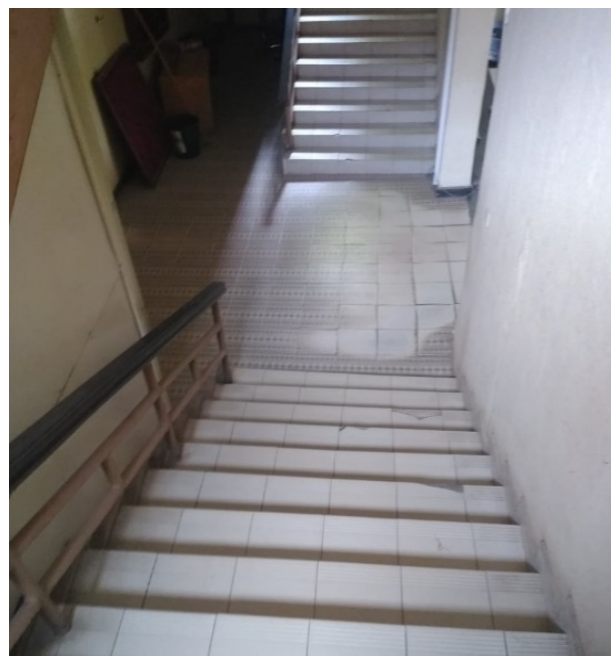
Figure 9. Staircase Flight Lobby
