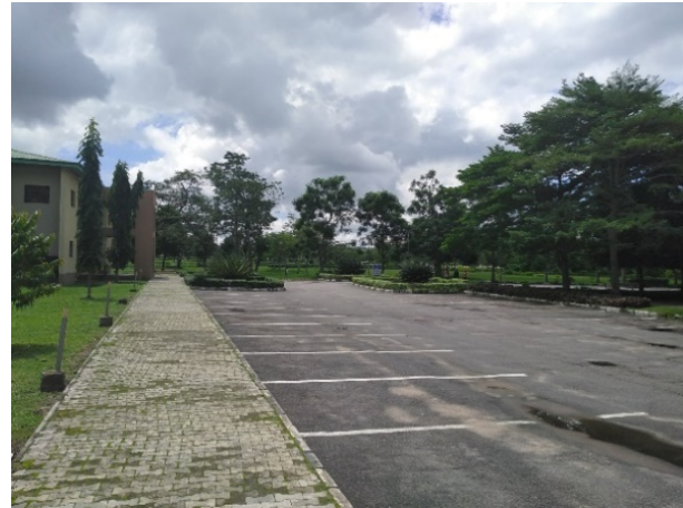
Figure 11. Side view of the Building with Adequate Vehicular Manoeuvring
