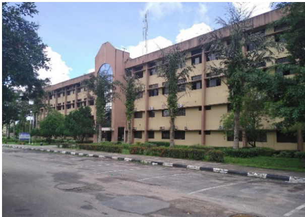
Figure 10. Front view of the Building with Adequate Vehicular Manoeuvring Space
