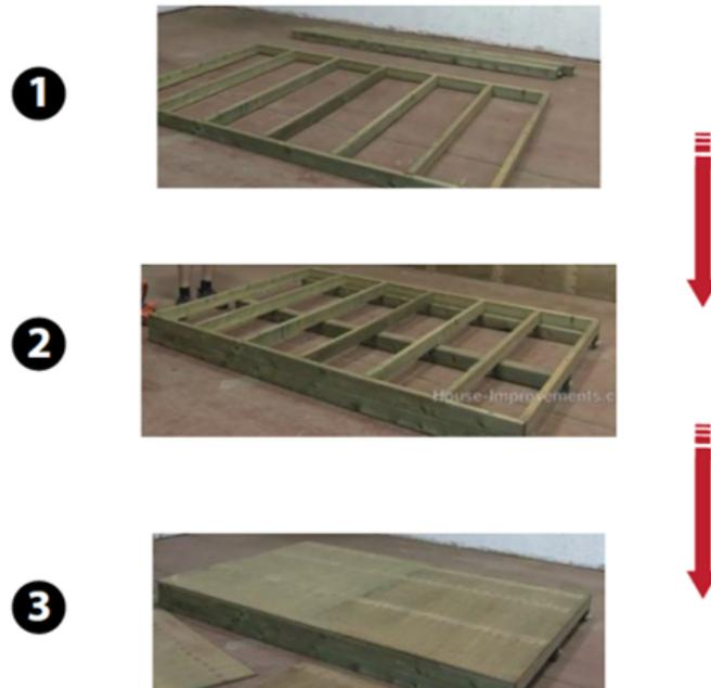
Plate 4.1: Process of Constructing the Timber Floor
