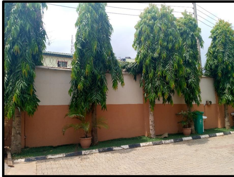
Plate 4.14 View of perimeter fence
