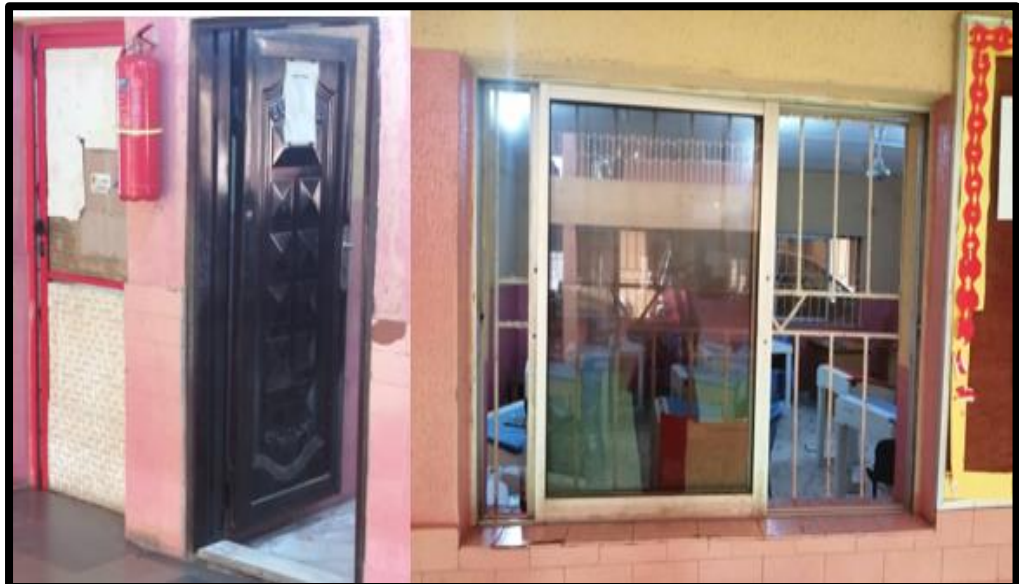
Plate 4.23 view of doors and windows
