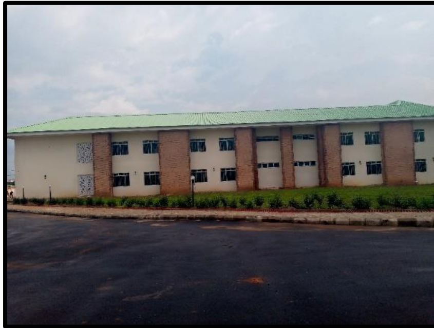
Plate 4.8 Windows facing the road for easy viewing
