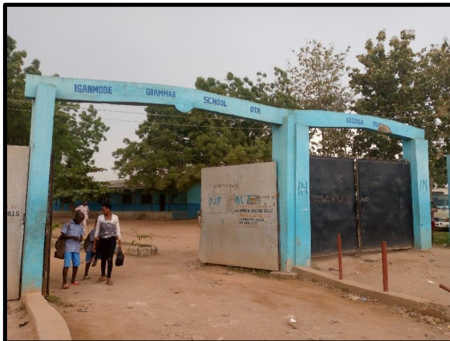
Plate 4.34 View of perimeter fence
