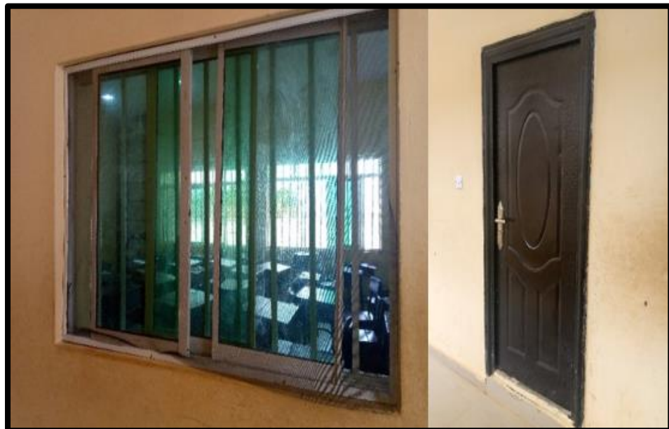
Plate 4.11 View of interior door and window
