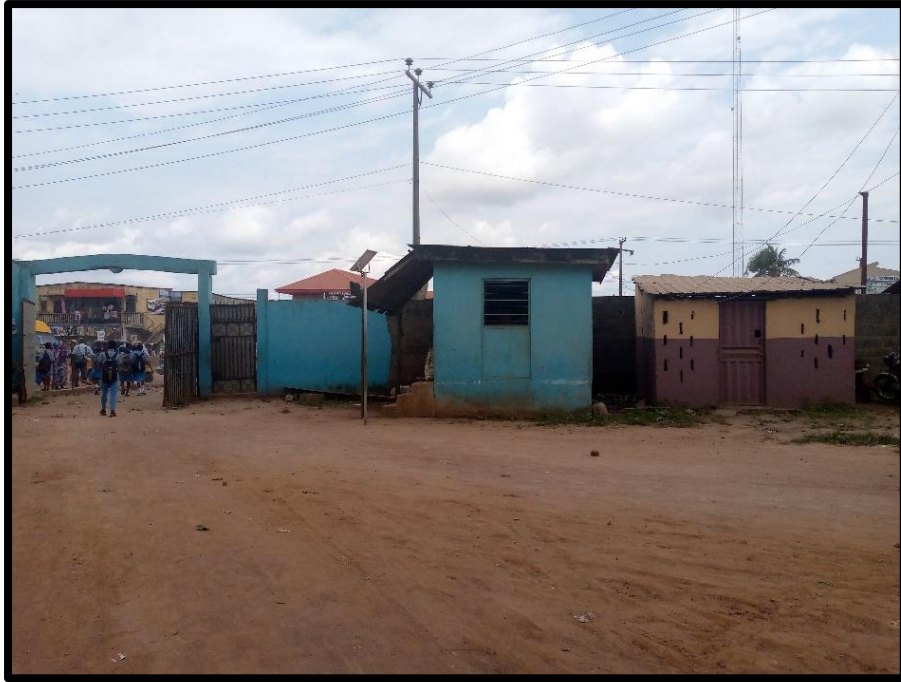
Plate 4.35 View of gate house
