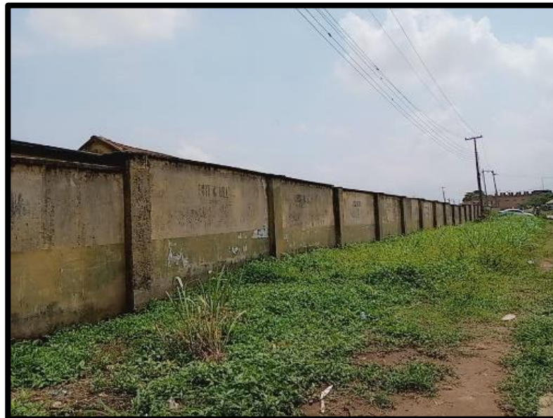
Plate 4.26 View of perimeter fencing
