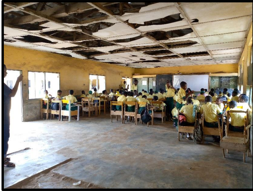
Plate 4.31 View of classroom
