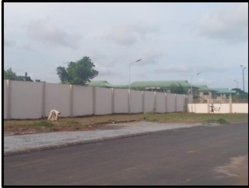
Plate 4.3 View of perimeter fence
