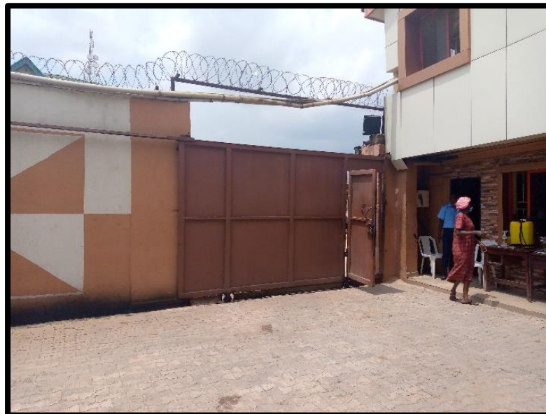
Plate 4.15 View of gate and gate house
