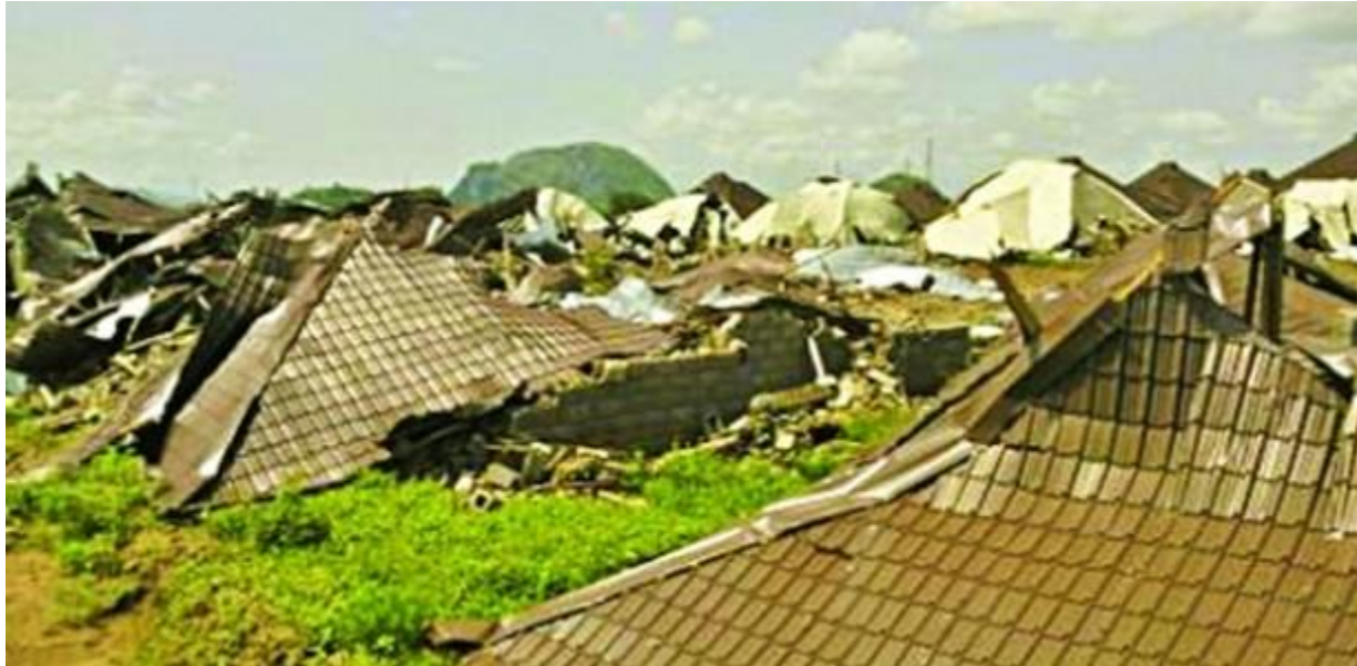
PLATE 1: A view of part of the demolished 500 housing unit in Abuja. (The SUN, 2012) [8].
