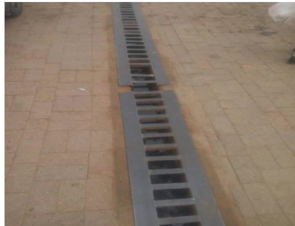
Figure 4. Stormwater pipe connected to a surface drainage at Justrite mall
