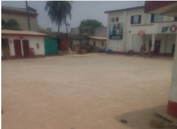
Figure 1. The premises of Grocery Bazeer mall with no drainage system for stormwater
