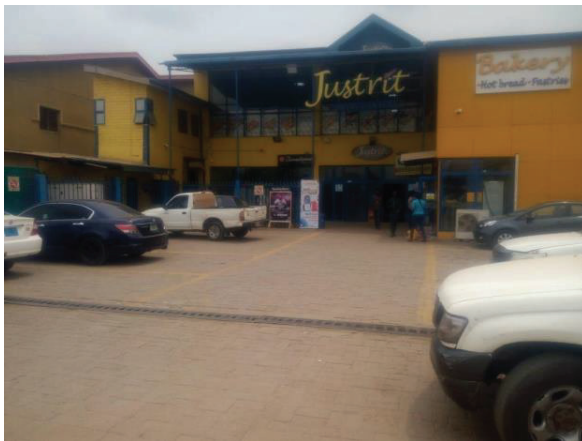
Figure 3. The approach of Justrite mall showing a covered stormwater channel at the carpark
