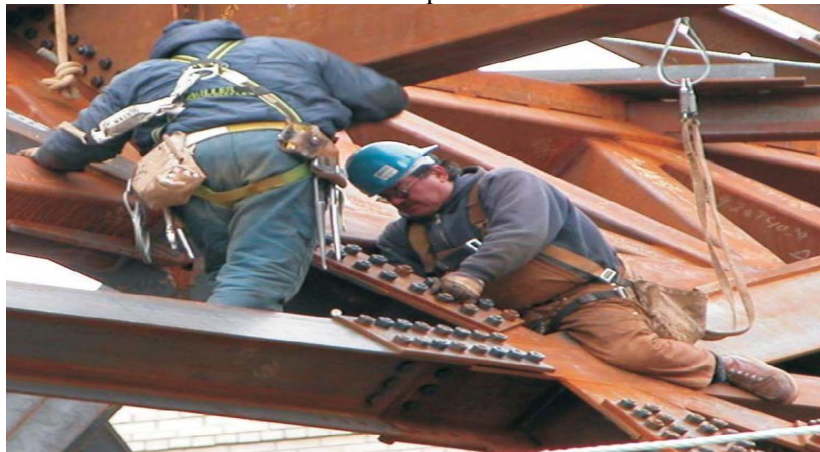
Plate 2. Bolted Connection used in Construction [11].
