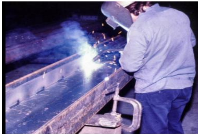
Plate 5. Welding of Plates [19].
