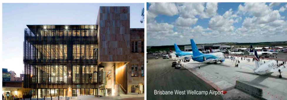
Figure 19. Global change institute building and Brisbane airport [12].
