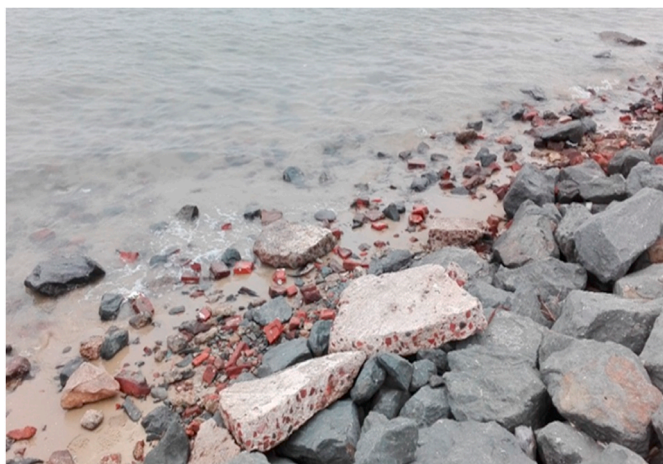
Fig. 2. Location of the concrete sample obtained from Durban Harbour (Maydon Wharf).
