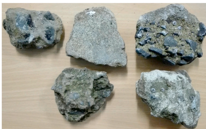
Fig. 3. Weathering and deterioration visible on the surface of the concrete samples obtained from Durban Harbour (Maydon Wharf).
