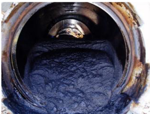
Fig. 2. Typical debris in a sour crude gathering and transportation system [39].
