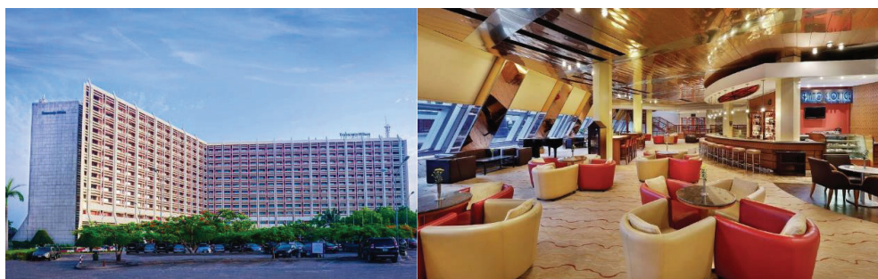
Plate 15 and Plate 16: Building Form and Interior Finishes
