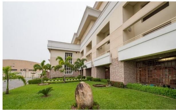
Plate 3. The roof and fa çade overhangs at the Rock Cathedral
