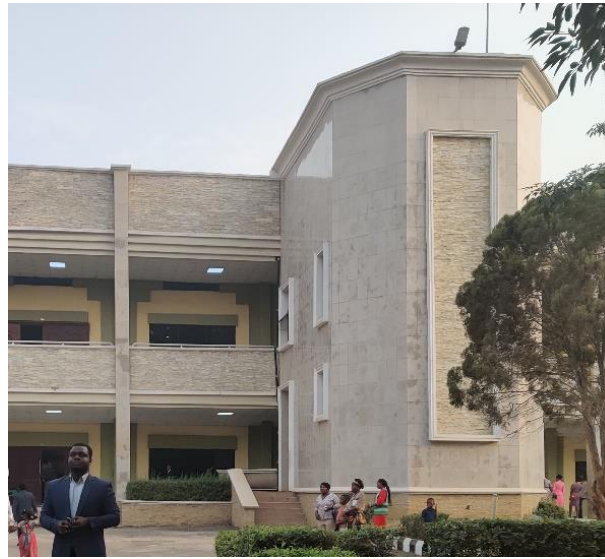
Plate 9. The stone and ceramic wall tiles cladding in Faith Tabernacle
