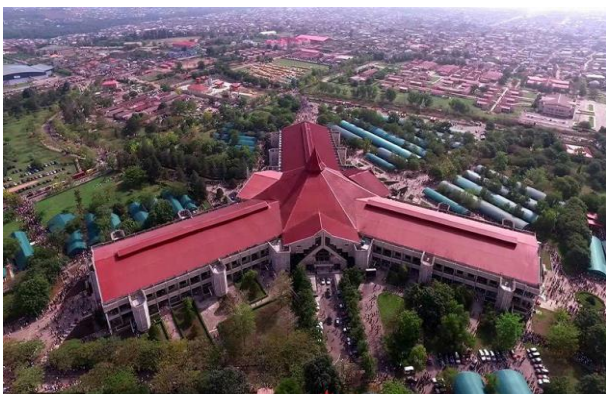
Figure 10. Aerial view showing the Faith Tabernacle (Source: Google.)
