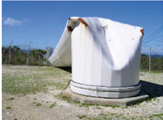
Fig. 8 Failed wind turbine tower during operation
