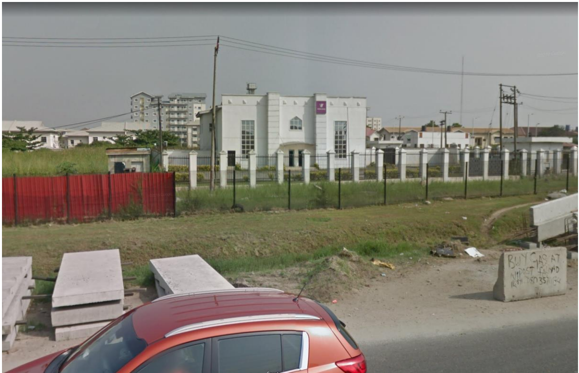
Plate 4.26 Adjoining development around the site (Wema Bank)
