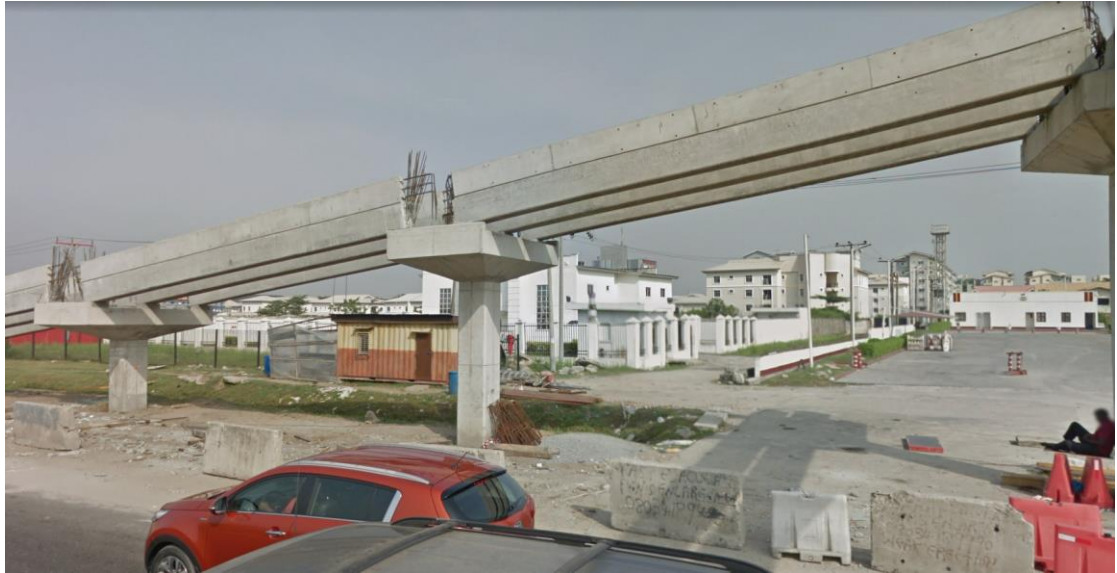
Plate 4.25 Adjoining development around the site (Wema Bank)
