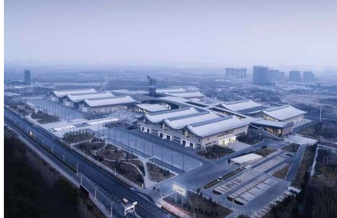
Figure 1: Aerial view of Shijiazhuang International Convention and Exhibition Centre
