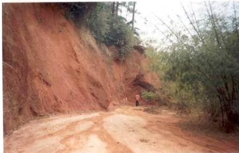
Figure 4. Gully side wall profile at Agulu Gully site.
