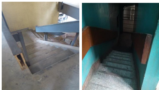
Plate 5. Stairs connecting different floor levels in building
