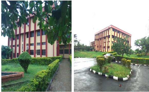
Plate 22. External Areas showing presence of walkway
