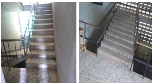
Plate 15. Stairs connecting different floor levels in building.
