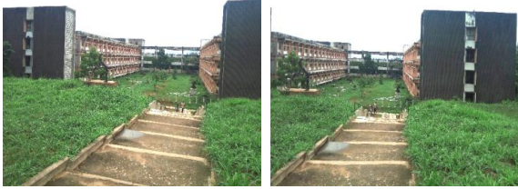
Plate 6. Pedestrian Access Route from Main Access Road
