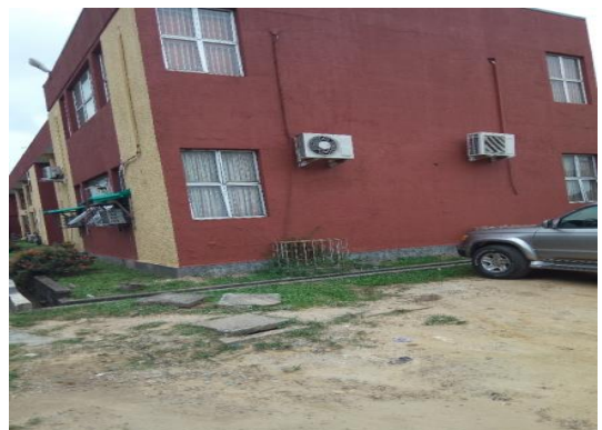
Plate 3. Areas left for car park around faculty buildings
