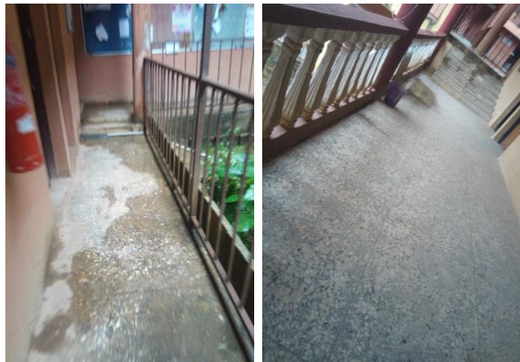
Plate 23. Internal veranda showing change in levels and steps used to navigate them
