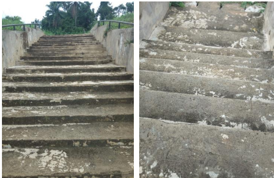
Plate 7. Pedestrian Access Route from Main Access Road
