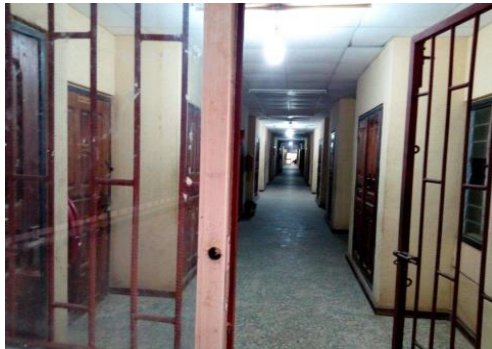
Plate 13. Internal Corridors flanked on both side by offices
