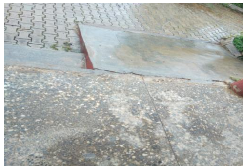
Plate 19. Ramps provided for main building
