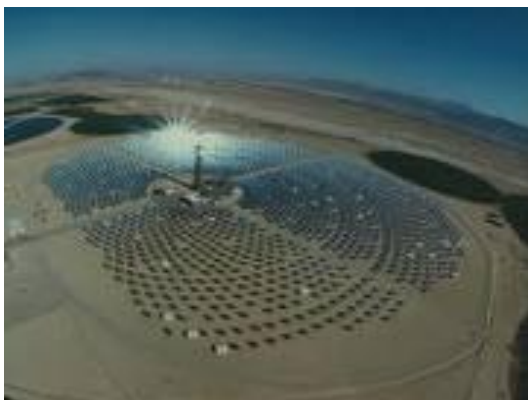
Figure 2.5: Heliostat (solar two)
