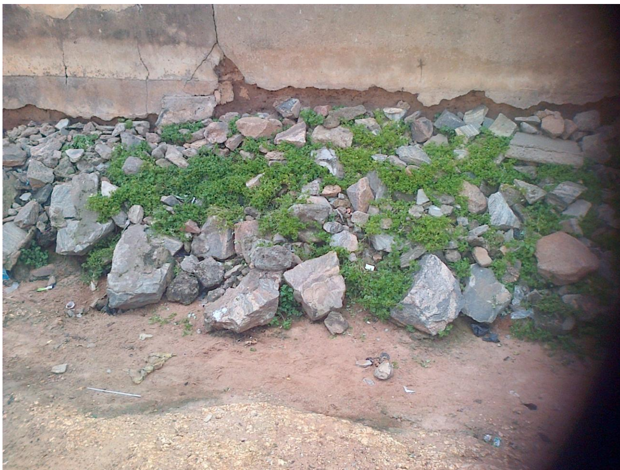
Plate 6: Local creativity in preventing further erosional impact on unpaved and ungreened open space around a building at Labo, Oranyan, Ibadan. Big boulders and rocks were used for this prevention. Consequently, green cover serves as prevention in addition to the stone used.
