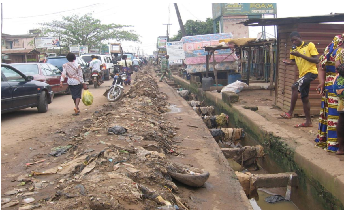
Plate 2: Large quantity of soil and other debris dug out of a drainage in Oju-Ore, Ota, a suburb of Lagos, confirming that unpaved and ungreened open space around buildings in the community generated large quantity of soil that were being washed away to the rivers and ocean.
