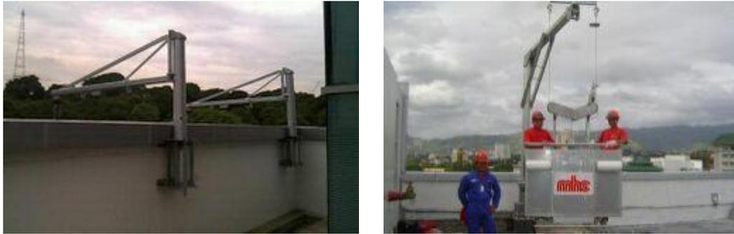
**Figure 3a&b: Rigging system**
