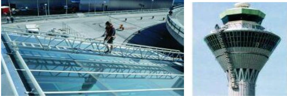
**Figure 6a&b: Ladder and gantry system**
