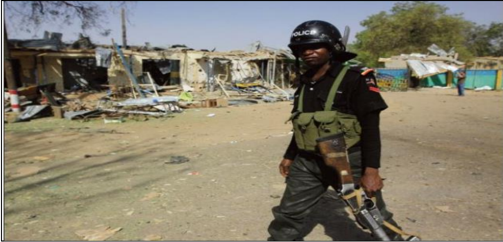
Figure 3: Bompai Police Barracks In Kano Destroyed During Ethno-Religious Violence
