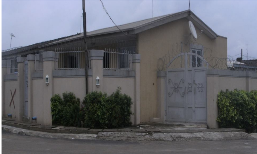
Figure 5 : Transformed house in The New Lagos Low-income Housing Estate, Surulere
