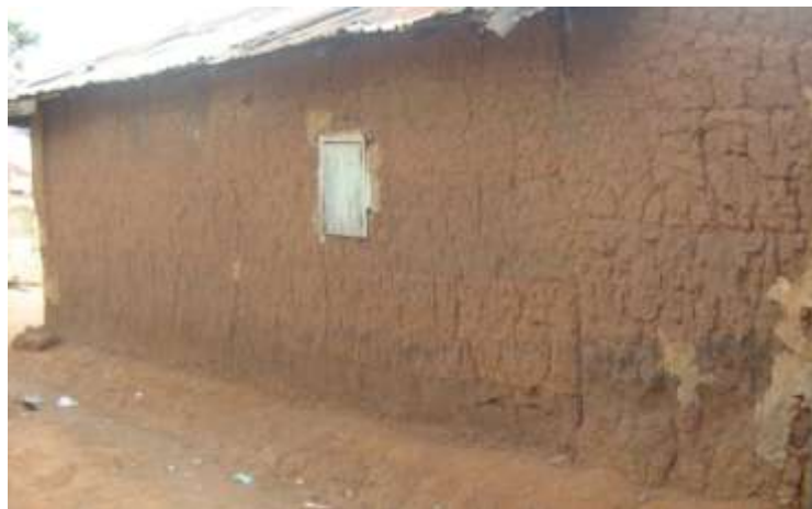
Plate 1: House Built of Mud Wall Technique
