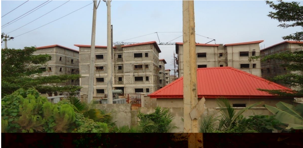
Plate 1: Igando Scheme Showing Wet Masonry Walls
