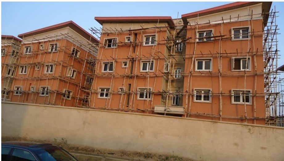
Plate 3: Sogunro Scheme I Showing Bamboo Scaffold
