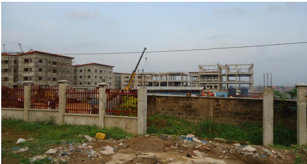
Plate 2: Igando Scheme Showing Hoisting of Precast Slab Panels
