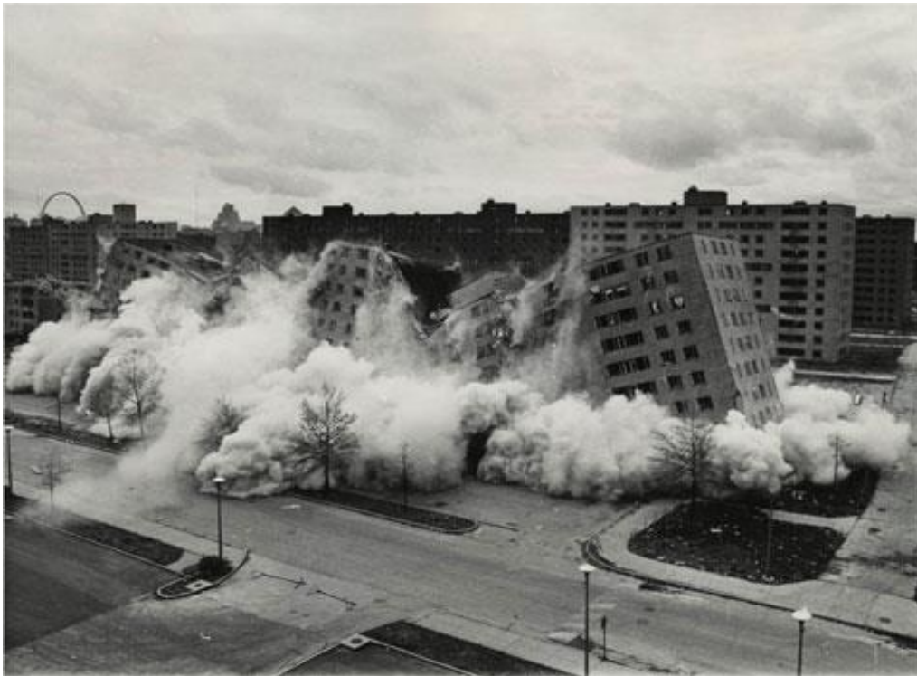
Figure (4) the demolition of the Pruitt-Igoe housing development
