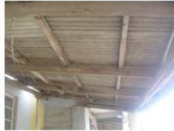
Plate 4.3.2: Roof Ceiling Showing Timber Trusses
