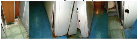
Appendix2: Picture of cracks in walls harboring microorganisms[13]
