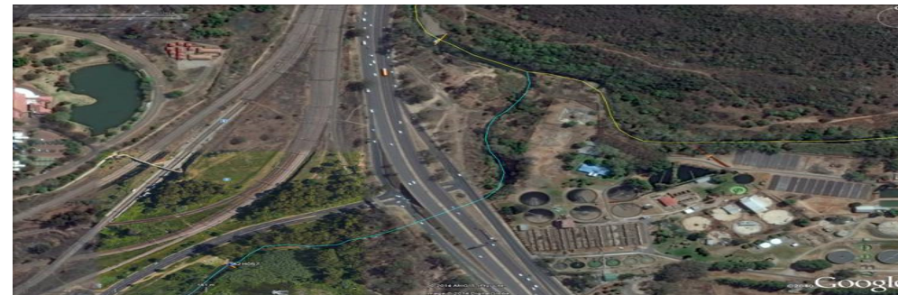
An aerial view of Daasport Wastewater treatment plant at close proximity to Skannerspruit stream
