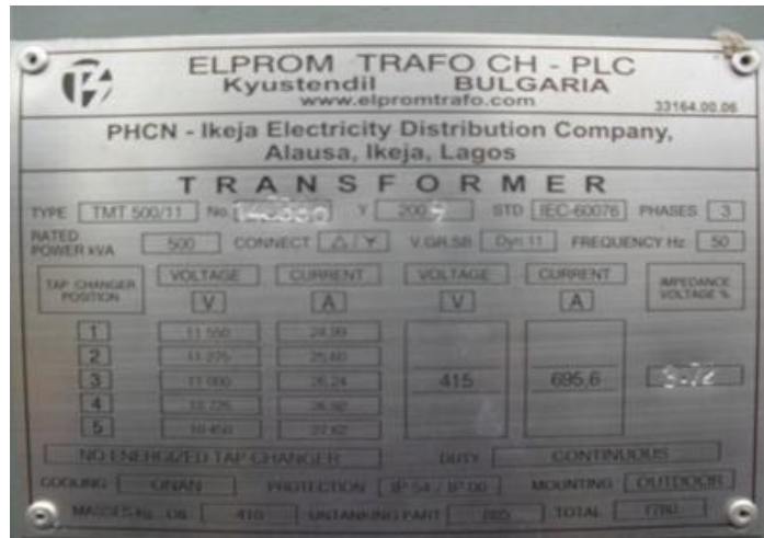
Figure 8: Transformer particulars
