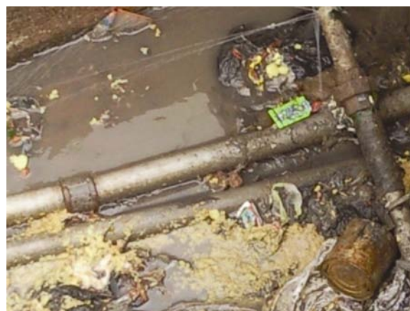
Fig. 1—Leaking water supply pipes lying in sewer 7
