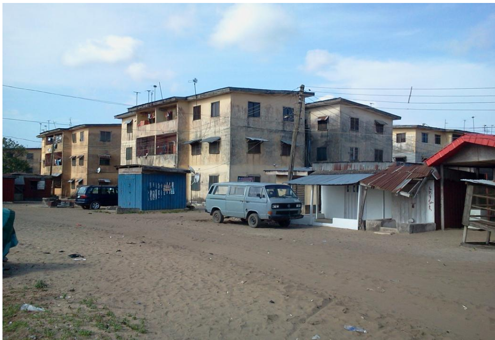
Plate 31: Iba Low Income (L.I.) Estate showing some of the blocks of flats (old) Source: Author's Fieldwork (2014)
