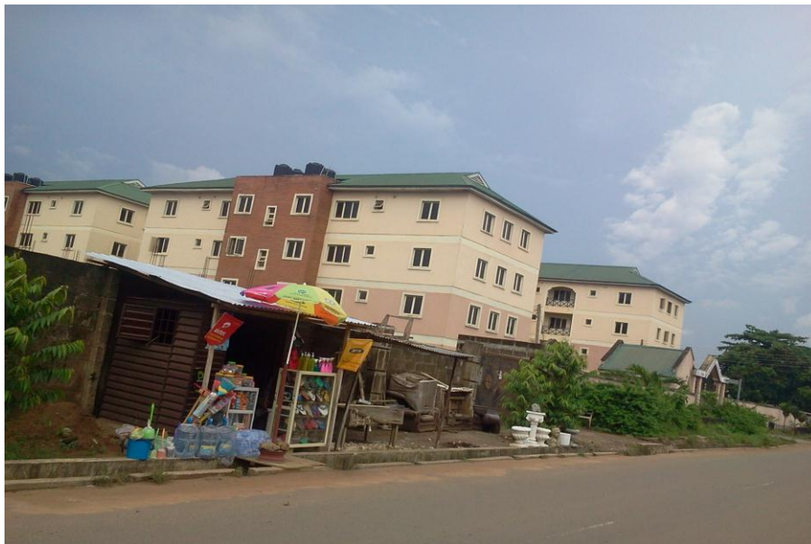
Plate 16: Ojokoro II Housing Scheme Estate1 blocks of flats, security block, and paved access road
