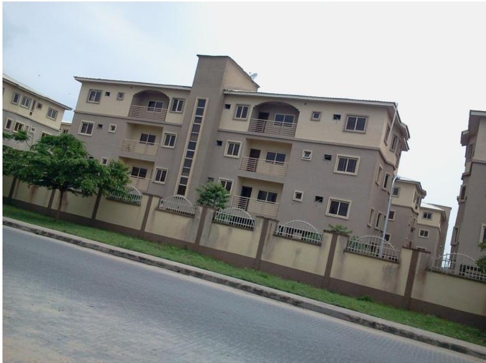
Plate 28: Cortex Housing Scheme showing 5 of the blocks of flats, Perimeter fence and paved access road Source: Author's Fieldwork (2014)
