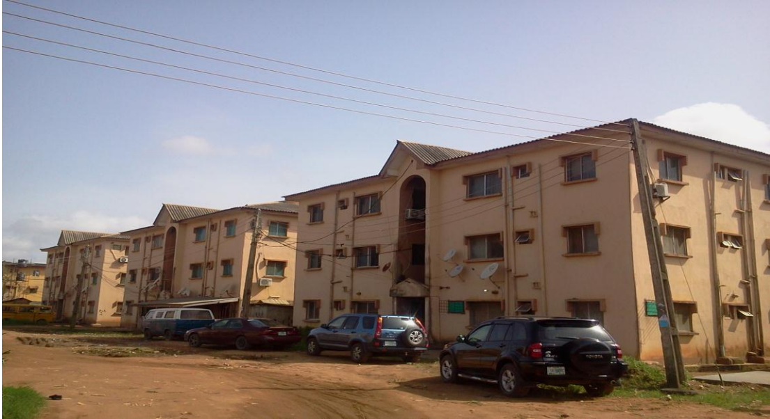
Plate 41: Isolo Low Income (L.I.) Housing Scheme showing 3 blocks of flats (A) and estate unpaved internal road Source: Author's Fieldwork (2014)
