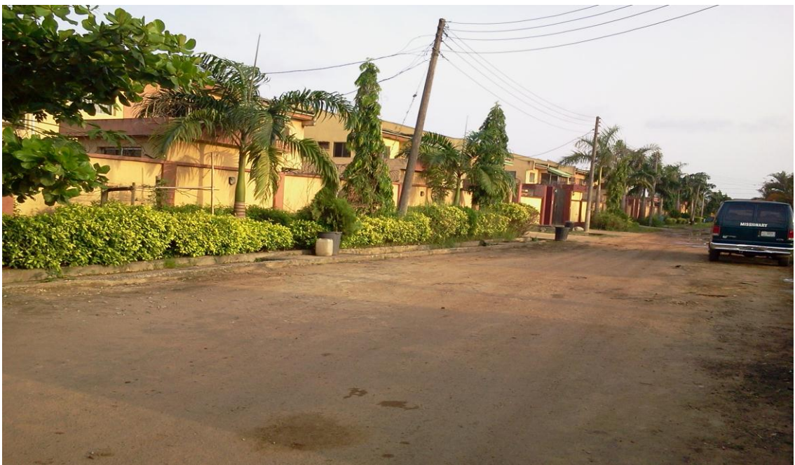
Plate 12: Satellite II duplexes and partially paved internal road with landscaped hedges and internal fencing Source: Author's Fieldwork (2014)
