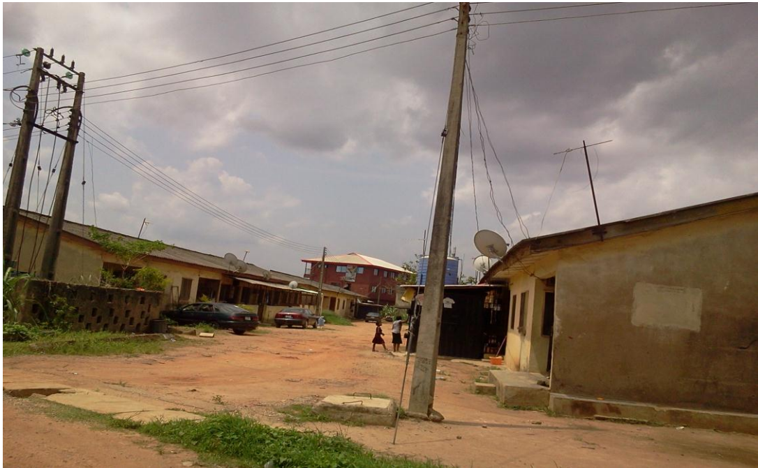
Plate 40: Abesan II Housing Scheme showing blocks of flats, unpaved internal road and transformer substation
