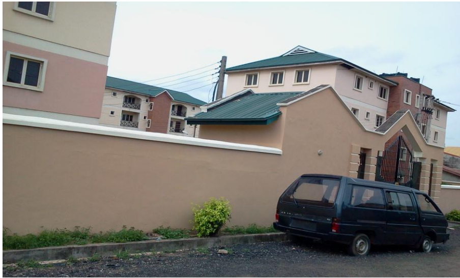
Plate 20: Iloro Housing Estate showing 3 of the 4 blocks of flats, security gate and fence Source: Author's Fieldwork (2014)
