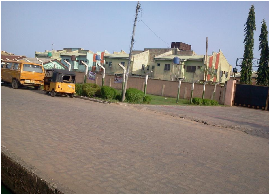
Plate 10: Satellite II duplexes and paved access road with estate fencing
