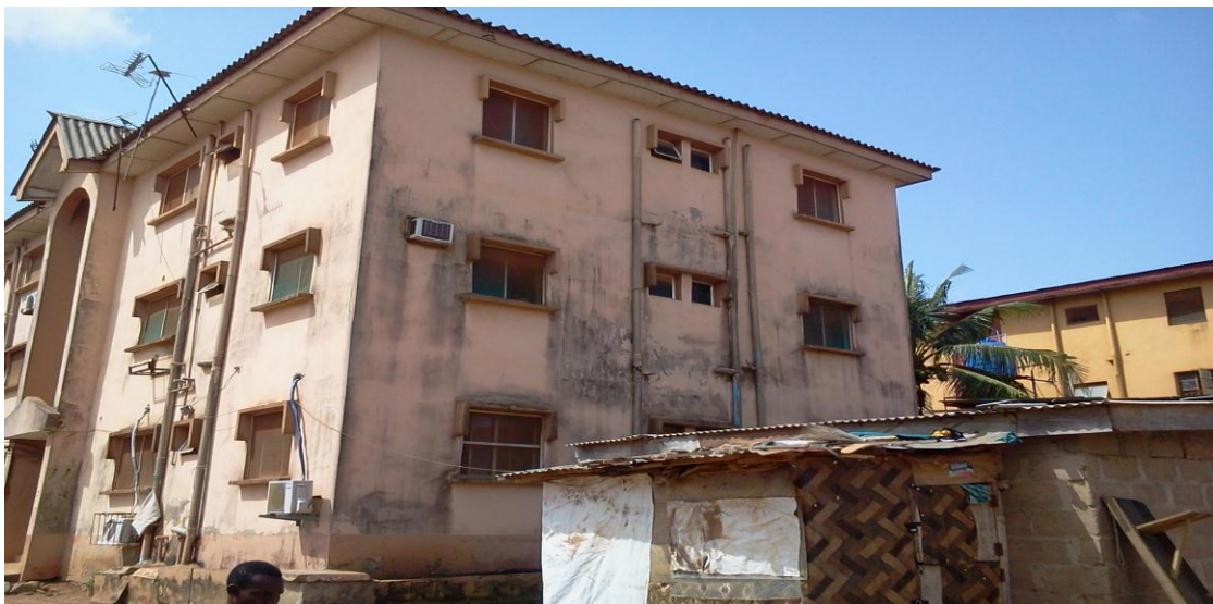
Plate 42: Isolo L.I. Housing Scheme showing 1 of the 2 blocks of flats (C) Source: Author's Fieldwork (2014)
