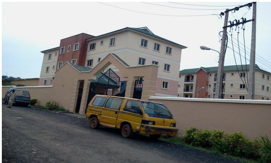
Plate 19: Iloro Housing Estate 2 of the 4 blocks of flats, security block/gate, and paved access road
