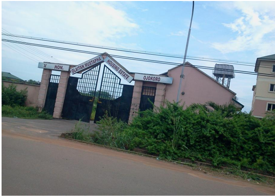
Plate 17: Ojokoro II Housing Scheme Estate2 security block, blocks of flats and paved access road Source: Author's Fieldwork (2014)
