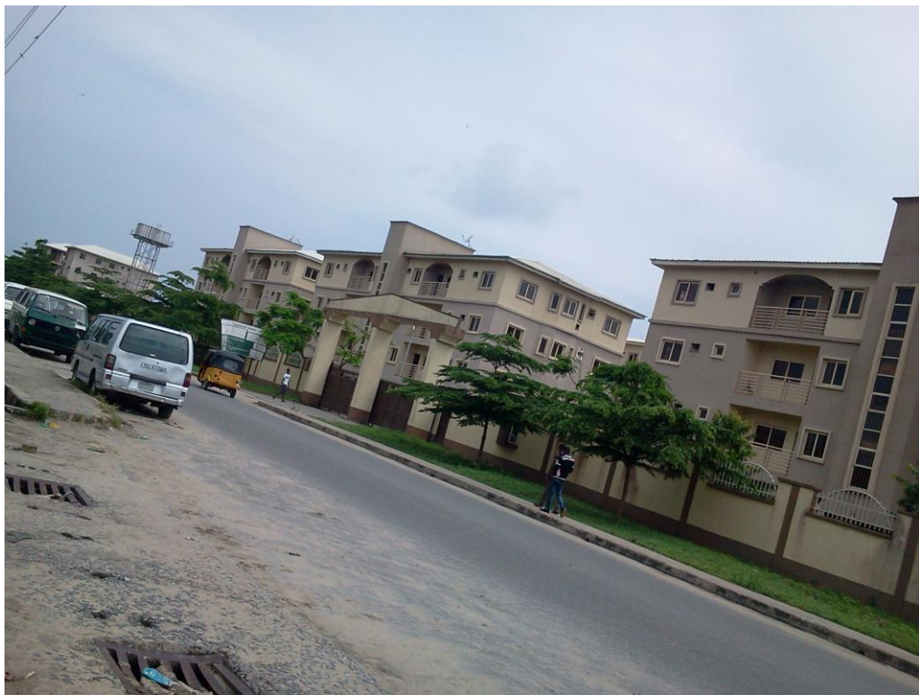
Plate 27: Cortex Housing Scheme showing 3 of the blocks of flats, perimeter fence/gate and paved access road Source: Author's Fieldwork (2014)
