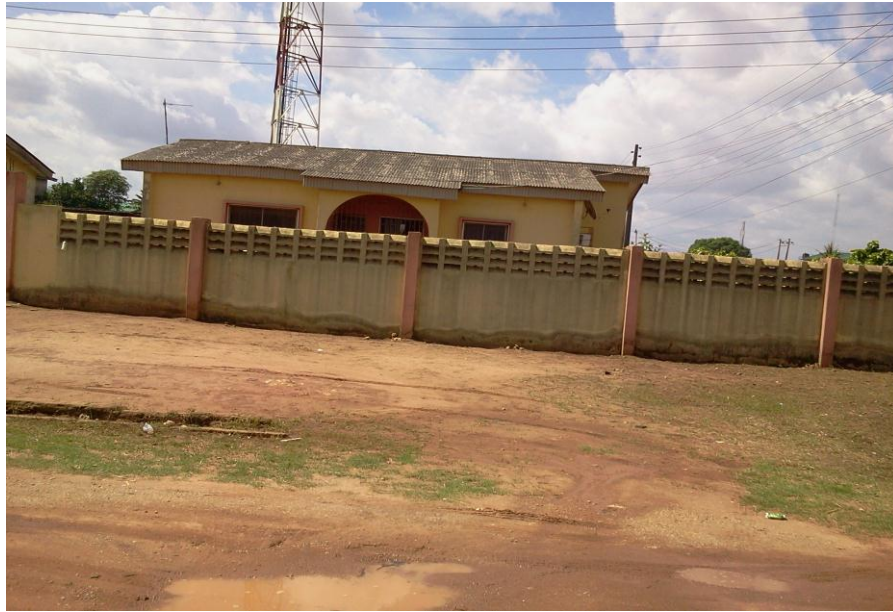
Plate 24: Abesan I Housing Scheme showing 1 of the bungalows, a property fencing and unpaved internal road
