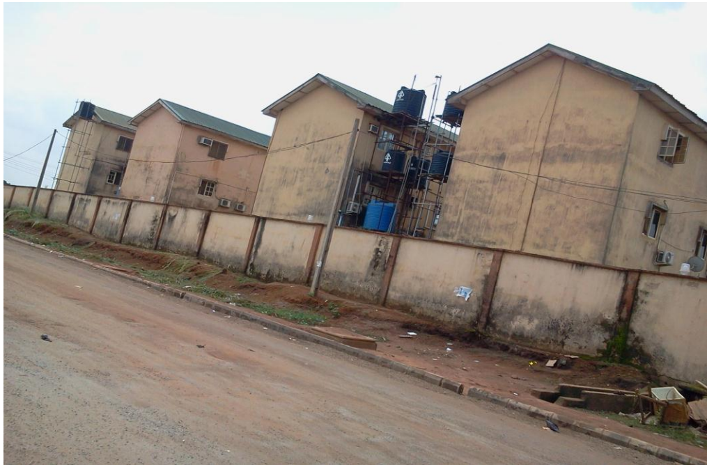
Plate 35: Millennium Housing Scheme Shasha showing blocks of flats and Perimeter fencing
