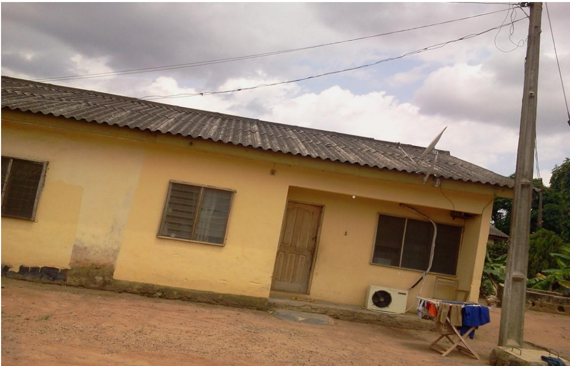
Plate 39: Abesan II Housing Scheme showing a block of flats Source: Author's Fieldwork (2014)
