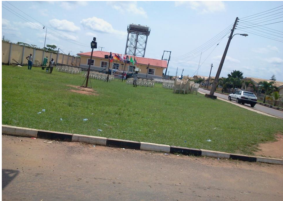
Plate 29: Diamond Estate showing administrative block, elevated water tank, some of the blocks of flats (right), perimeter fence (left) and paved internal roads Source: Author's Fieldwork (2014)
